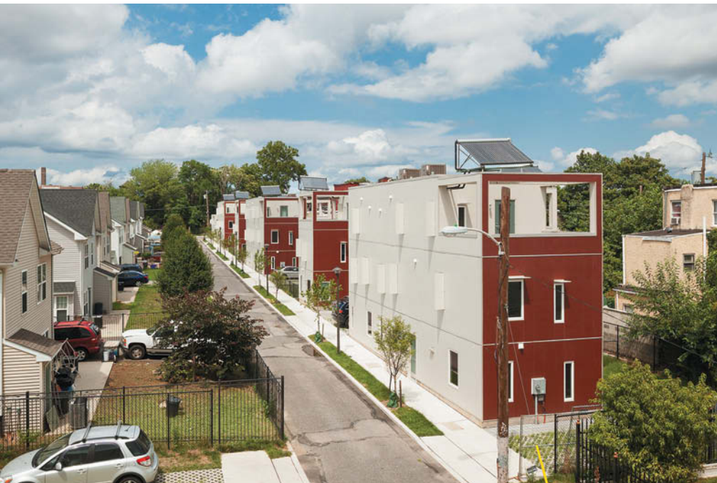
A block of green affordable housing on Sheridan Street developed by Asociacion Puertorriquenos en Marcha. Designed by ISA.
