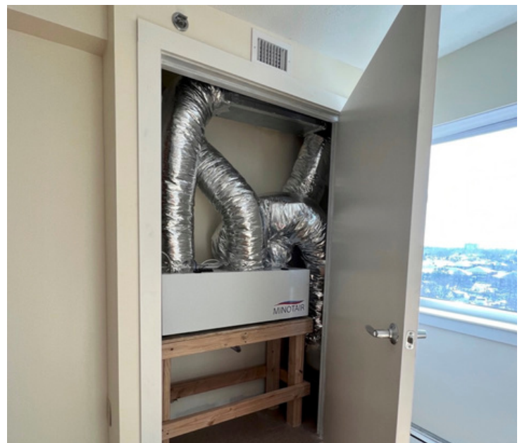
A Minotair heat pump and heat exchanger was installed in a new mechanical closet on the outside wall of each apartment.
