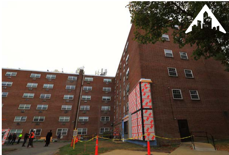
Fairweather Apartments, Salem, during a panel installation demonstration.
