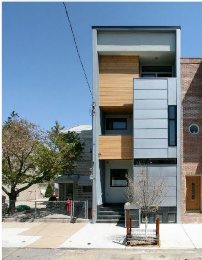
THIS PAGE Berks Rowset by Onion Flats reimagines the idea that row homes should be next to each other by connecting them at the back. The cisterns two separate facades sit opposite sides of the street.
