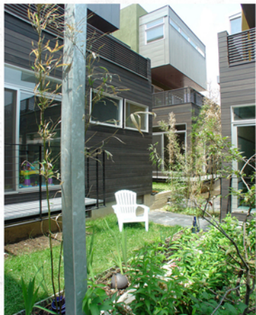
The houses surround a courtyard garden. There is space between the units, and bays and terraces project from them.
