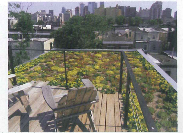
OPPOSITE European design inspired the ground-breaking water management system at Rag Flats LEFT Permeable paving outside of Thin Flats ABOVE Green roofs harvest water on the firm’s projects
