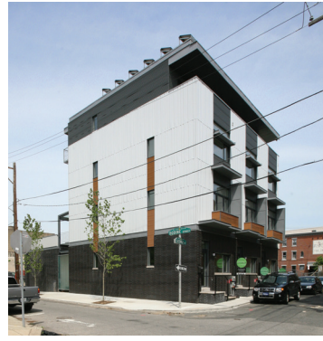
figure 14.15: Photo of completed Phase 1 of Stables Townhomes
