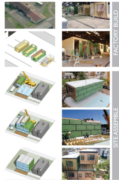
figure 14.7. Process of modular from the factory to site assembly
